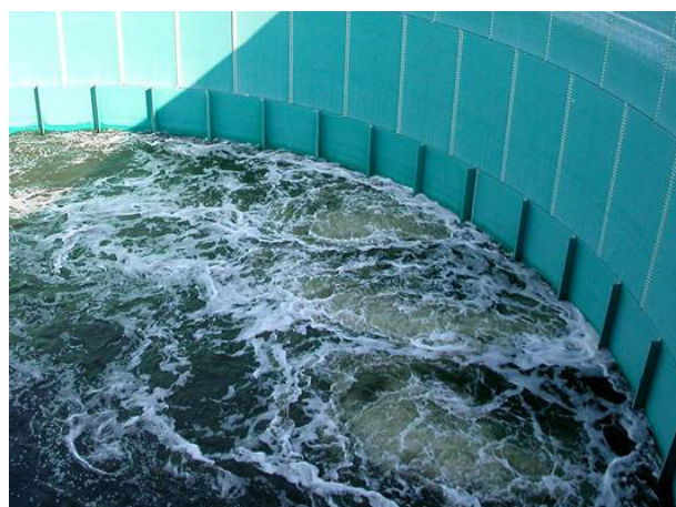
An aerator with chopper pump and ejector system provides simultaneous aerating and mixing. | All images courtesy of Landia Inc.
