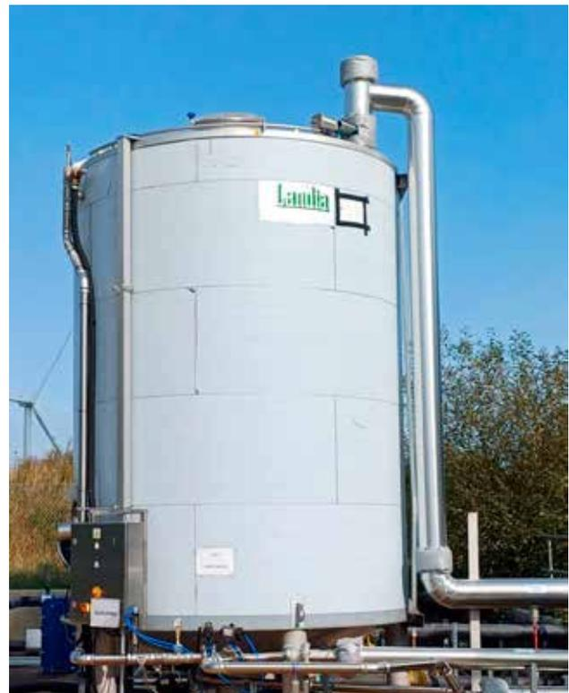
At the end of the process, in order to meet the legal requirements of a feedstock that contains animal bi-products, there are now two (25 m<sup>3</sup>) Landia pasteurisers, which heat the final effluent to the required temperature of 70 °C.
